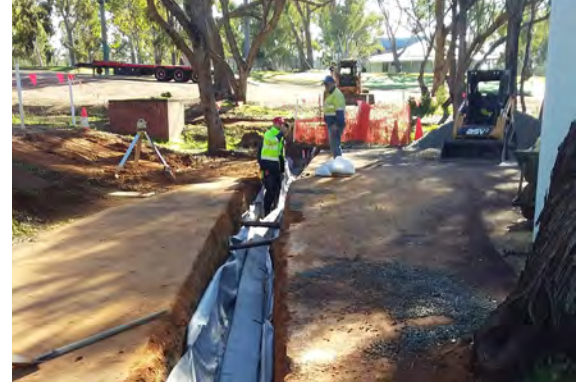
Sub-soil drainage
