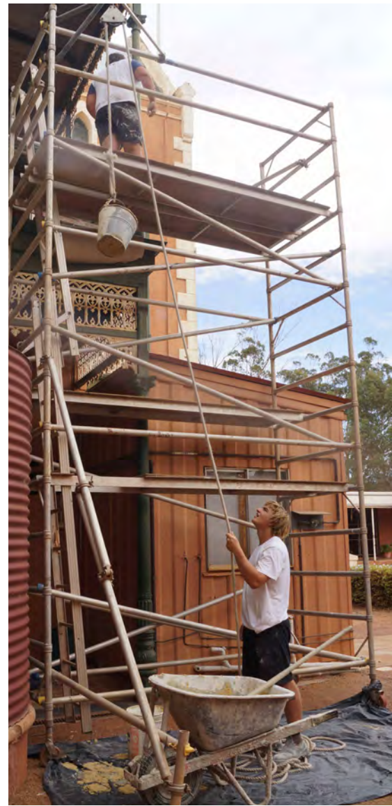
Getting the render up to the 1 st level of the College
