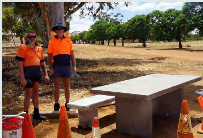
Shady and Stephen installing one of the tables
