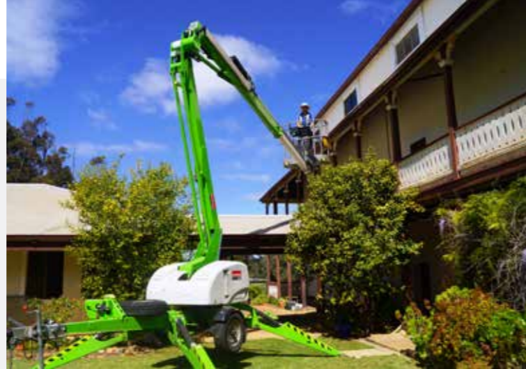
Replacing gutters at the Monastery
