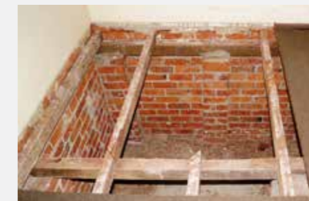
The lift shaft during construction
