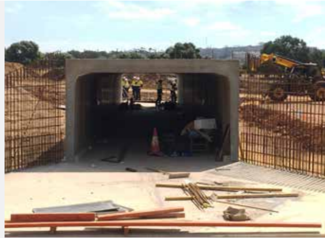
Livestock underpass being built
