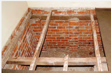
The lift shaft during construction
