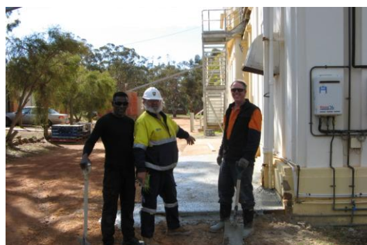
Sumith, Steve and Taffy (Decmil) laying concrete!
